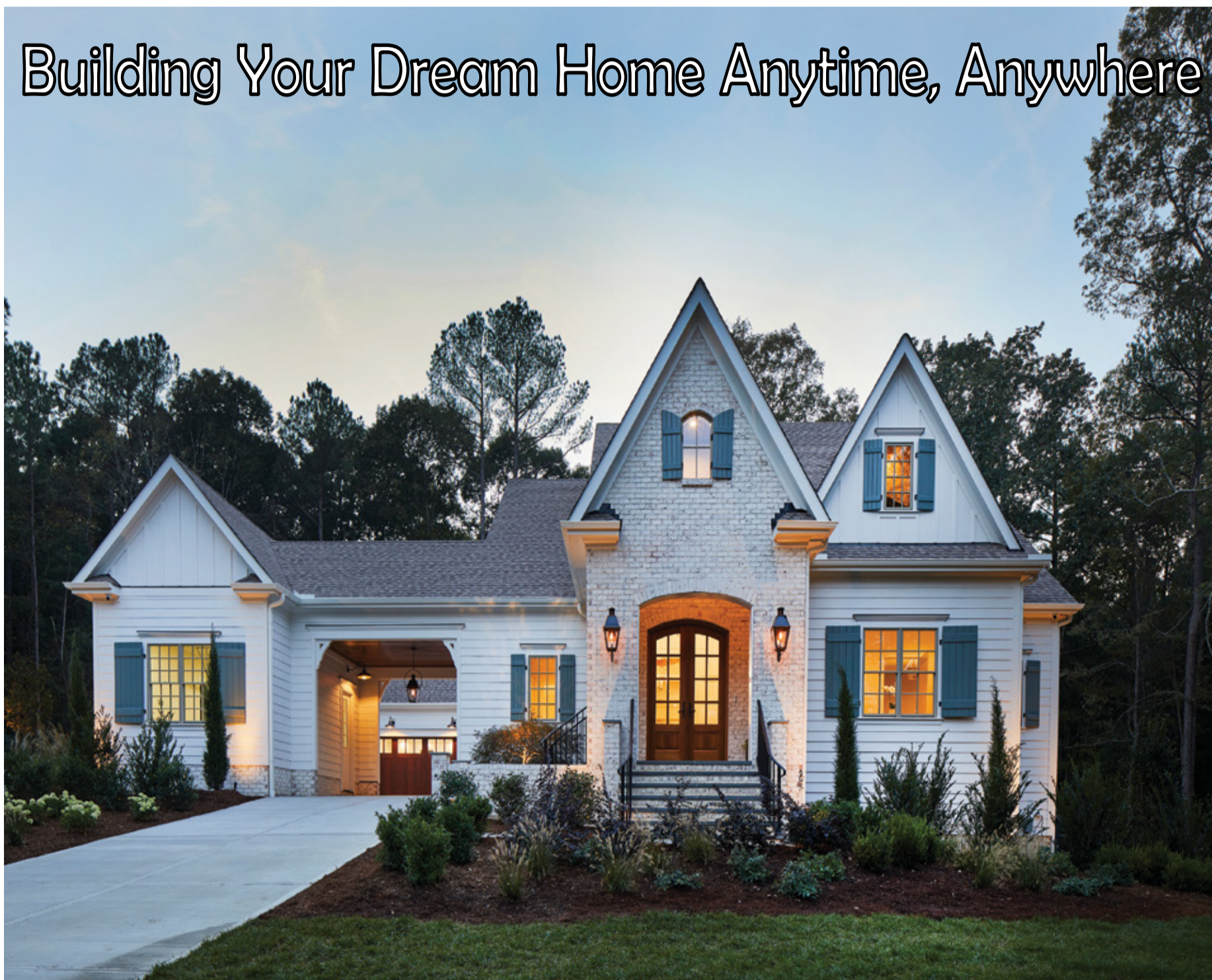
Photo courtesy of Laury Glenn and Paragon Building Group
