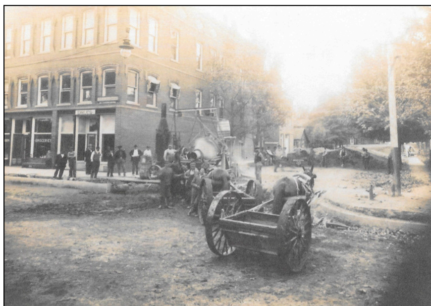
None of the towns had paved streets in the early days, and traveling on a dirt street or road was especially difficult after a good rain. In 1916 Darlington decided they had had enough and bricked Main Street. It remained as a brick street until the early 1960s.
